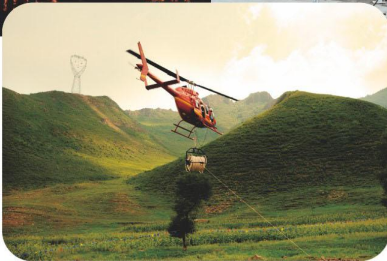
Solution for helicopter stringing of overhead line construction
